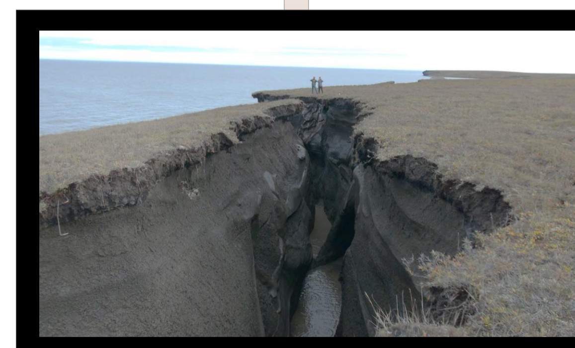
Fig.7) A large block failure on Pelly Island in 2016.
